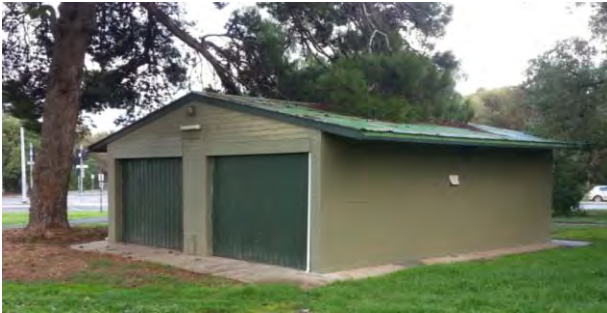
Existing Maintenance Shed
