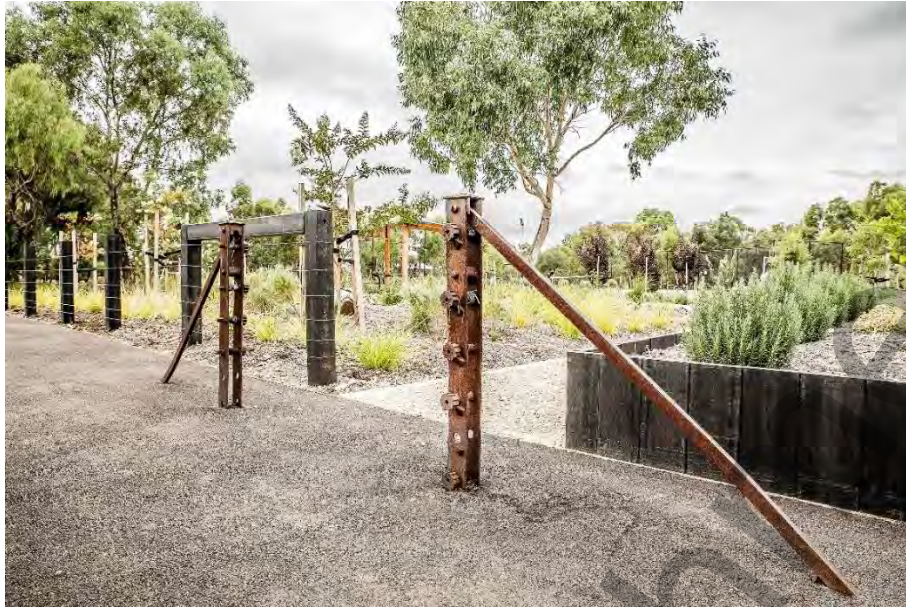
Wrought Iron Gate Posts on Mackinnon Parade
