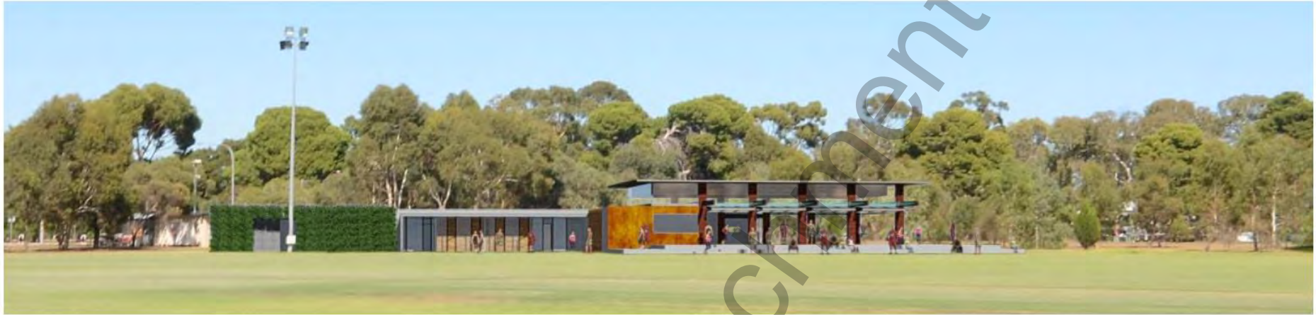
View from East (Oval & Mann Road)
